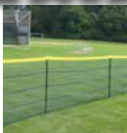
4. Place poles & sockets in holes.
