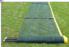
5. Roll up fencing with poles in place.
